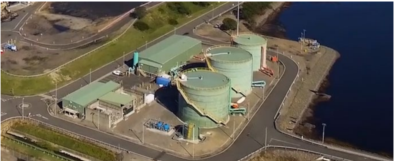
Figure 2: Remineralisation Plant Installed Onsite (shown in foreground in front of larger tanks)
